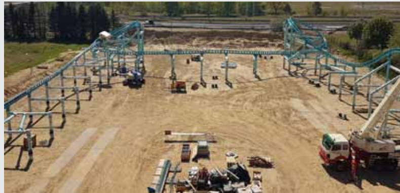
Announced last October as the world's longest roller coaster at sea, on board the Global Dream, the test setup for Space Cruiser by Dream Cruises has begun. This will be the highlight of 'Dream Park at the Pier', the very first theme park at sea. The first photos of the construction process show the scope and scale of the offshore roller coaster.
